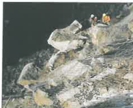
Photo: de filets pare-blocs.
